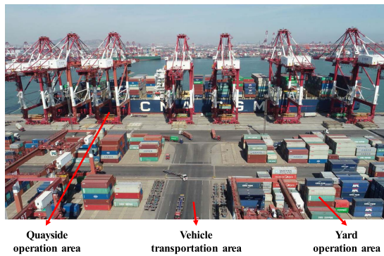
Fig. 1. Real layout of ACT: Take Qingdao Port in China as an example.
