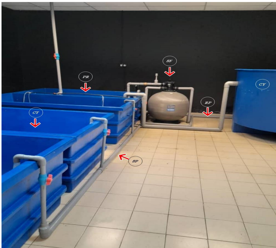
Figure 4.5: The phytoremediation unit showing the mechanical filters and Caulerpa tanks of IMTAS.
