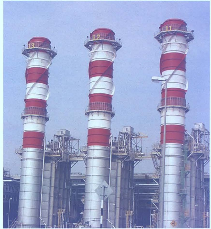
Petroleum industry in Kerteh Ölindustrie in Kerteh
